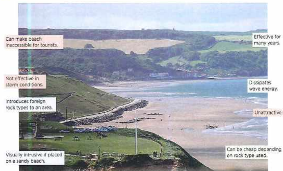
Figure 2.20 Rip rap are large rocks placed in front of a cliff; these are below a landscaped cliff at Whitby in Yorkshire.
