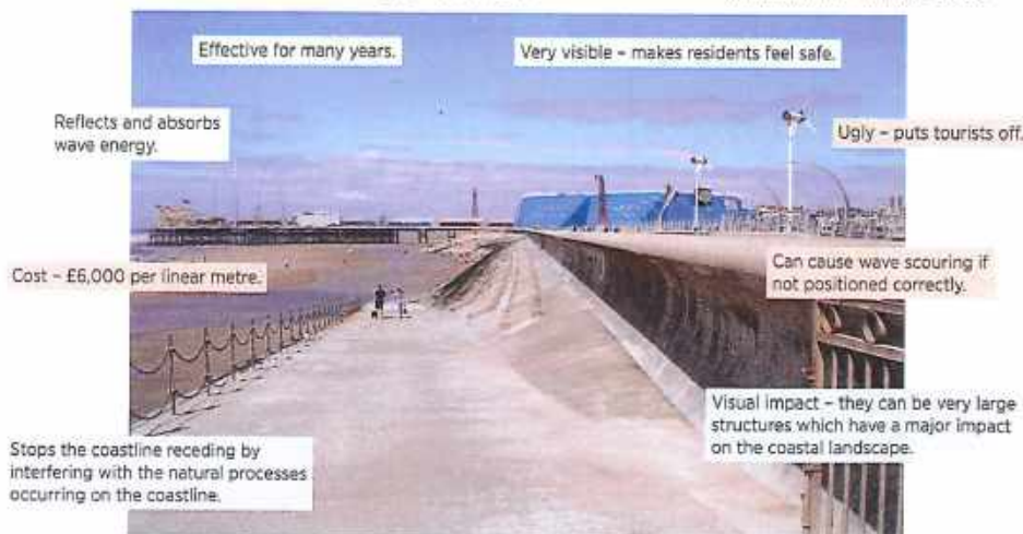
Figure 2.18 Sea walls are usually made of concrete; the newer ones have a recurved top, like this one at Blackpool.
