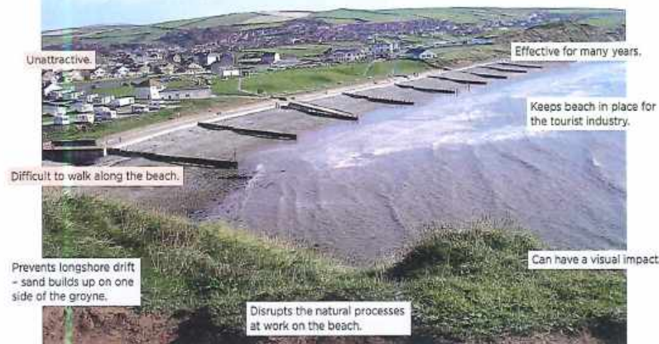
Figure 2.19 Groynes are usually made of rock or wood like these at St. Bees in Cumbria; they stretch from the coastline into the sea.
